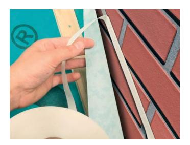
Bands or tapes offered by FAKRO are used for durable joining, sealing and repairing roofing membranes and non-permeable underlays. They eliminate the risk of water penetration into the insulation and rafters through holes formed as a result of puncturing the membrane with pliers and roofing nails. They are also recommended for attaching membranes and underlays to structural elements such as wood, wall or metal. They seal gaps around windows, light tunnels and chimneys.
