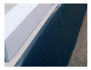
EUROFLEX systems are used for anti-moisture insulation of foundations, terraces, ceilings, roofs and floors. With special embossed areas, it forms a gap to allow additional ventilation of insulated surfaces. The system consists of:
